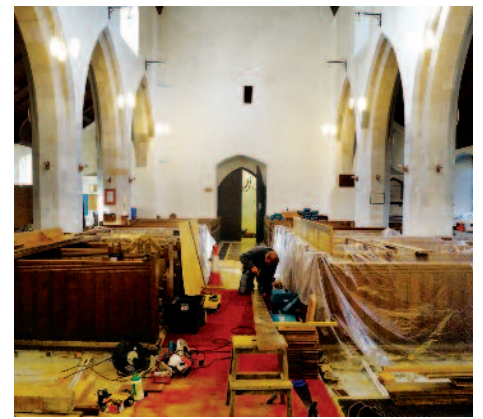
Building works, St Bartholomew's Church Lostwithiel
